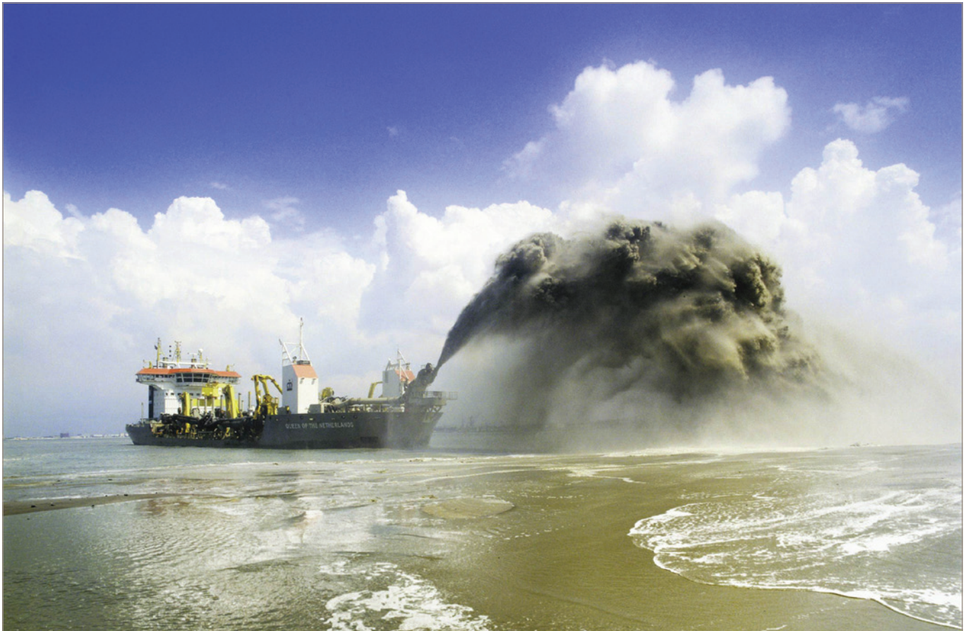
Figure 4. Beach nourishment will protect the North Sea coast as well as reclaim land for future use
